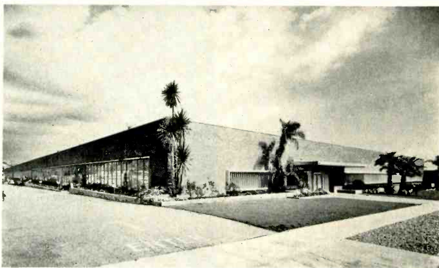
Electro Data's new computer facility in Pasadena, Calif.
