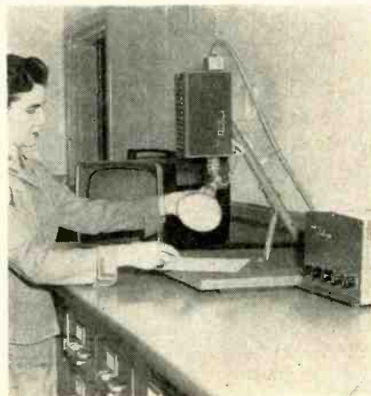
Closed-circuit tv camera, installed in the bookkeeping department of the Bank of Belmont, North Carolina, links the main building with its new Glenway drive-in branch, located 100 feet away. As shown above, requested information from the files is placed under the camera for transmission to RCA portable receiver in branch.
