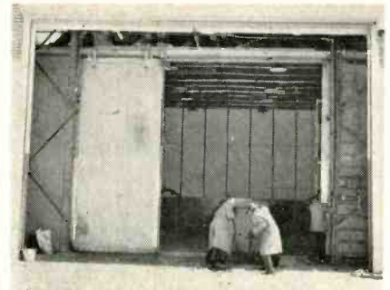
Looking through the large equipment door into the shielded room
